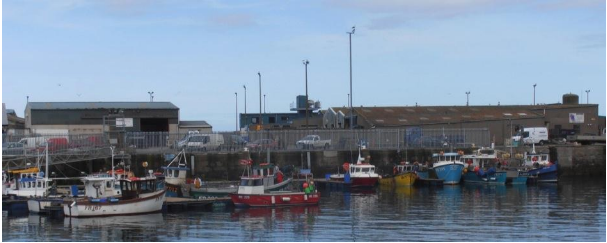
Figure 25. Main harbouring facilities at Peterhead for under 10m vessels, access via a ramp to floating dock, to cope with the high tidal range (authors own photo)
